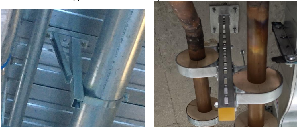
Figure 6 Cantilevered post bracing
